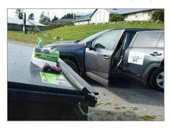
Figure 25. Installing chains with carabiners and instructional decals on Hitacu bins
